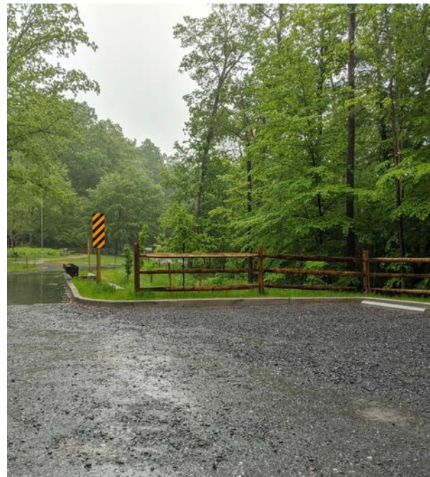
Trail parking areas should be designed to compliment the natural character of their surroundings. Features such as wood rail fences, pervious paving, timber bollards delineating no parking zones, and natural landscaping can formalize parking areas without detracting from the surrounding character.
