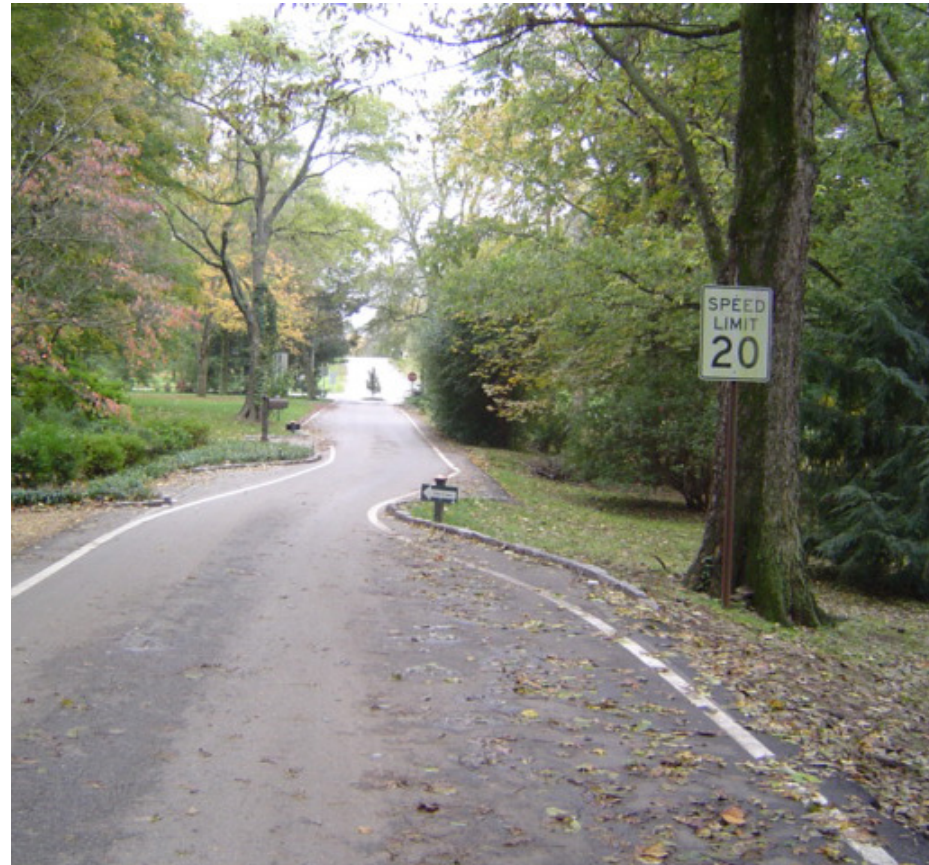
Low-cost alternatives to improve safety on local streets include removing center striping and replacing with reflective edge lines (left) and traffic calming techniques, such as chokers, designed to reduce the speed of vehicles.
