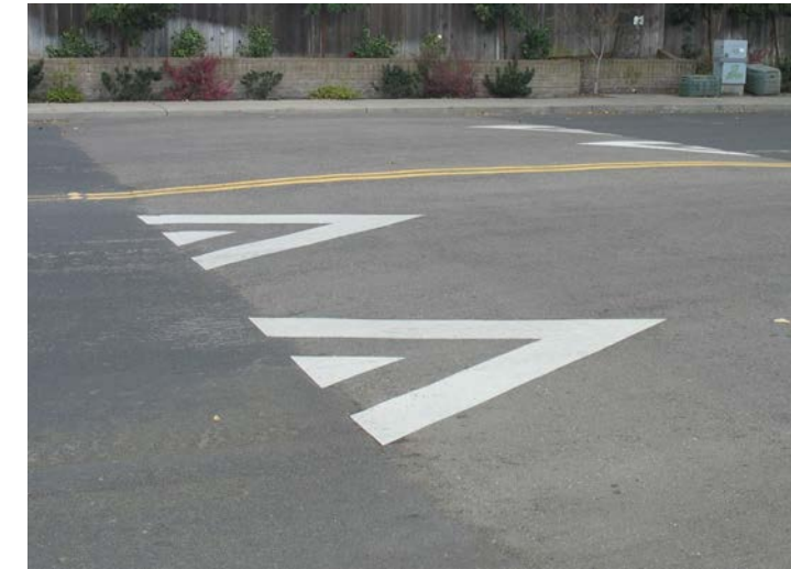
Examples of engineering applications that can curb dangerous driving behavior include rumble strips at pedestrian crossings (above, left), gentle-rise asphalt speed humps (above), and speed cushions (left). These traffic calming applications have evolved over the years to address issues such as emergency access and forcing near stops at each instance. It should be noted that drill down speed cushions allow bikes and strollers to utilize the gap along the roadway edge. The asphalt style of speed humps have a very gentle slope, so impacts are minimal.
